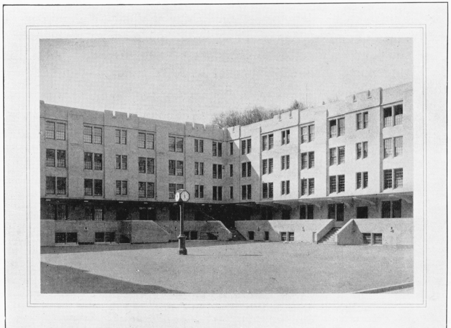
New South Barracks, looking at the hollow square. This structure is fitted throughout with Scovill Flush Valves.
